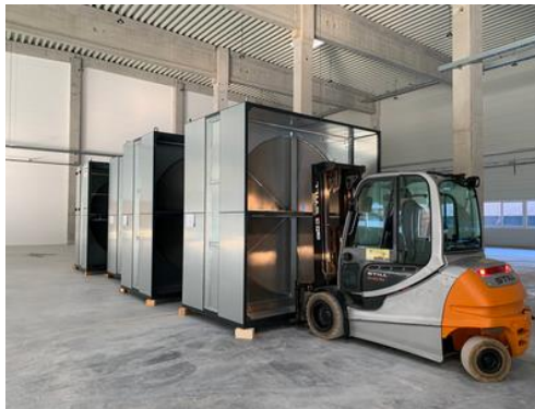
Delivery of sustainable heat exchangers to reduce energy requirements in the new finishing center.
